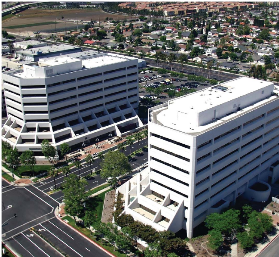
Sandpointe South Coast Metro complex holds aerospace firm's HQ
